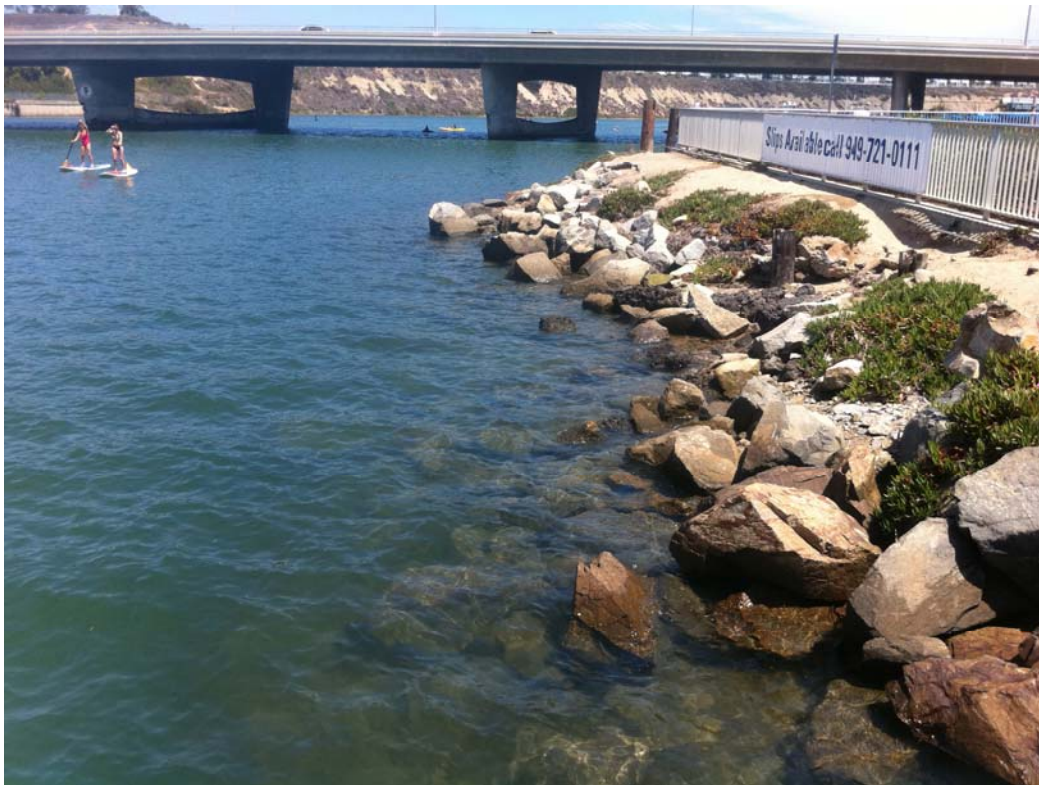
Figure 3a. View of Project Area Shoreline Facing North
